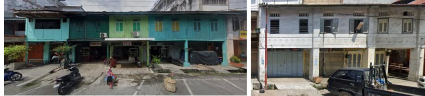
Figure 10. (a) shophouse with wooden materials on the second floor, (b) shophouse with brick material on both floors
